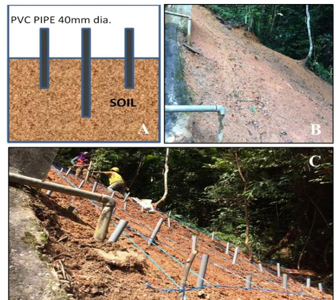
Fig. 3: Installation of PVC pipes for grouting
