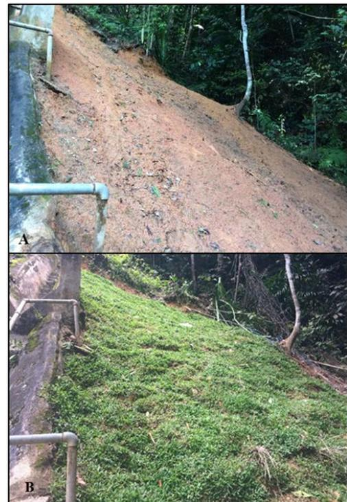
Fig. 7: A) Study area showed eroded surface B) After vege-grout treatment, study area showed growth of grass covering the top-soil
