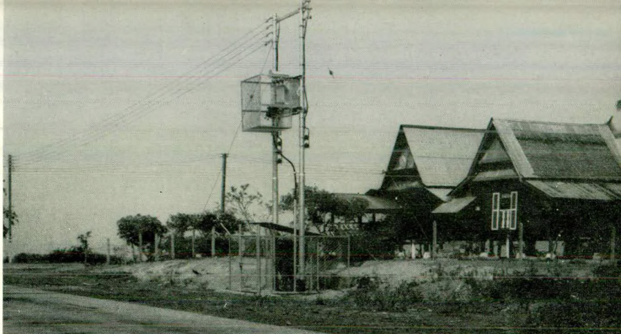
A Rural Scheme — 50 kVA Pole Mounted sub-station at Pantai Kundor with a typical Kampong house in the back-ground.
