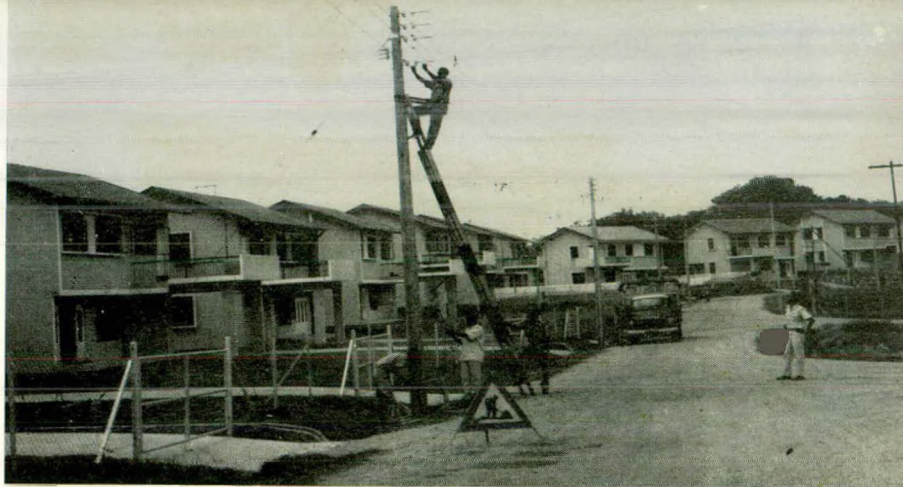
Erection of L.V. mains at Sentosa Gardens a Housing Estate of Stately Bungalows at Bukit Baru, Malacca.
