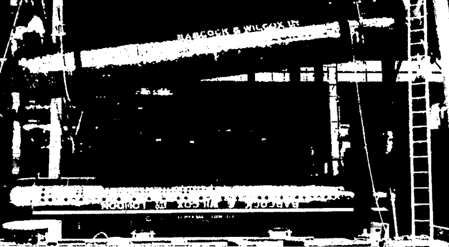
Malacca Power Station— Final Extension Lifting of No. 4 Boiler Steam Drum.
