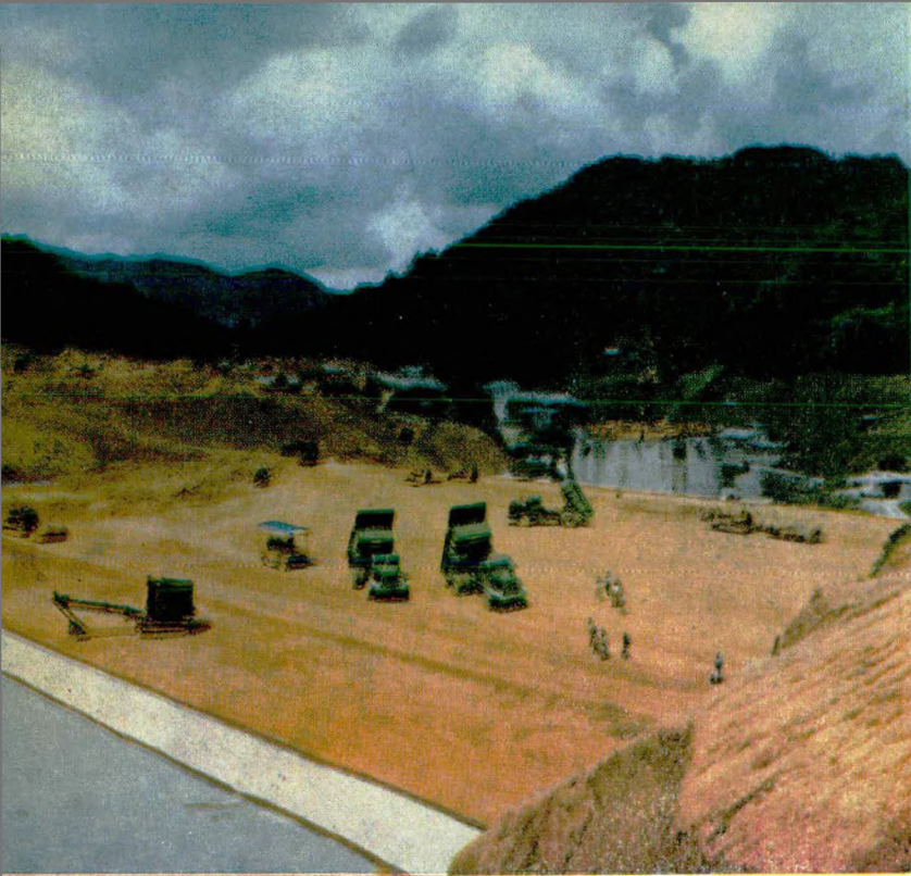
Placing earthfill in Jor Dam.
