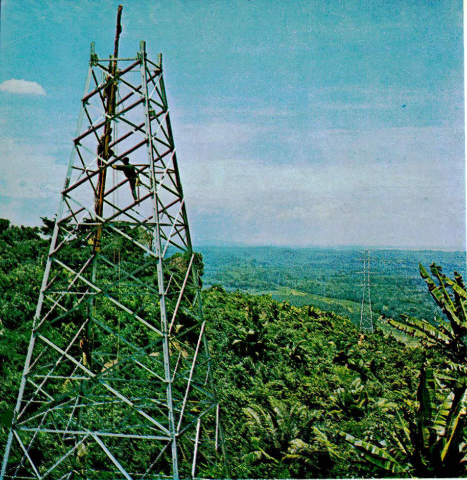
132 kV Transmission Line Tower Erection near Woh.
