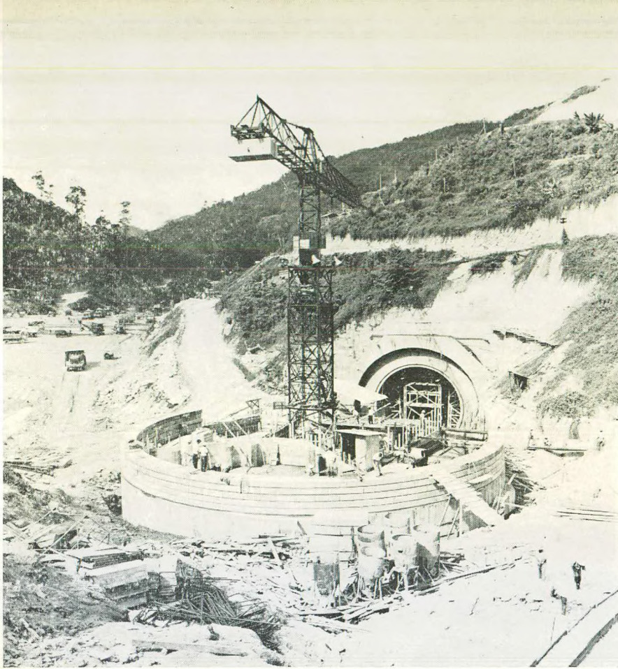
Jor Dam Siphon Bellmouth Spillway. — Blockwork commenced — upstream. Portal of Spillway Tunnel in background.
