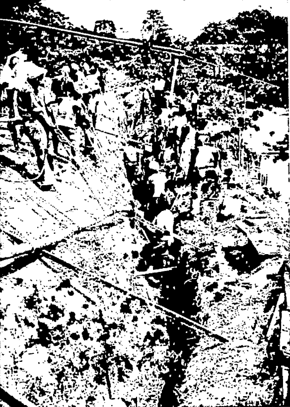
Rescuing a 33 kV cable from the ravages of the Sungai Kroh, Kuala Lumpur.
