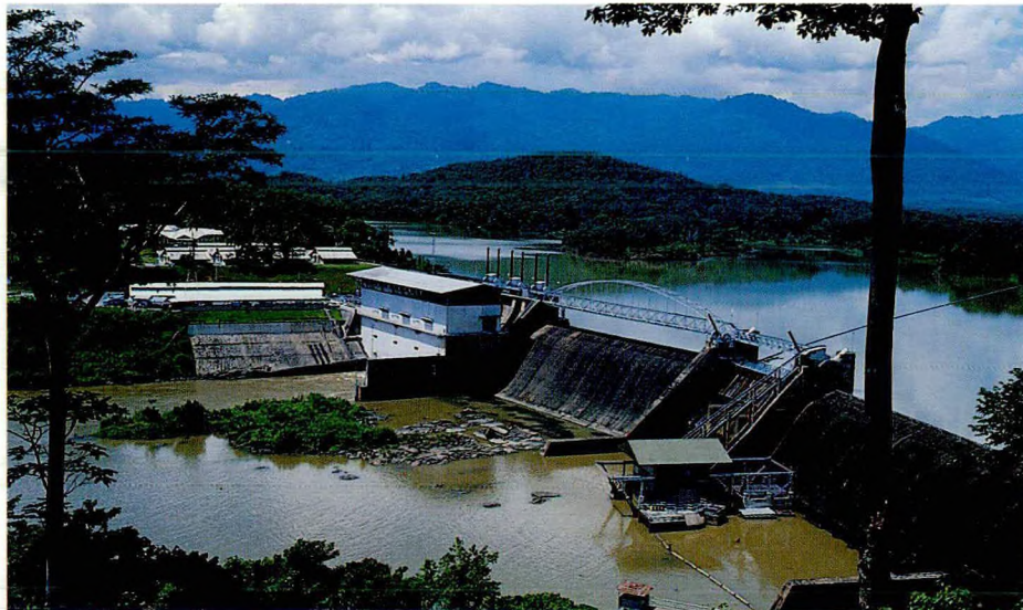
Pemandangan di Stesen Janaelektrik Chenderoh. A view of the Chenderoh Power Station.
