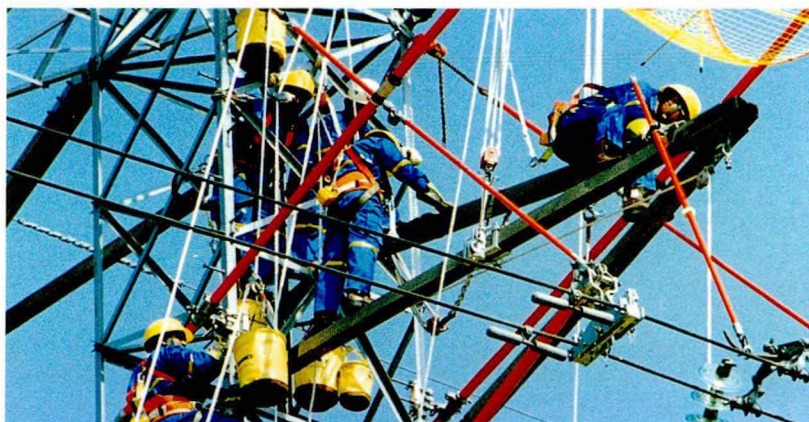
Live-line maintenance work in progress.
