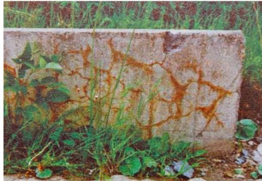
Fig. 1. Map cracking due to ASR deterioration on a concrete wall [2]
