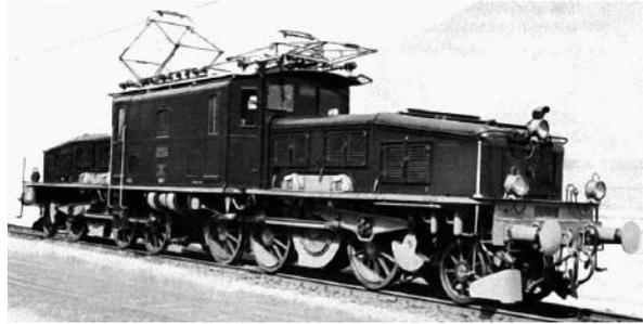
*Fig. 1.4: SBB Ce 6/8 II for single-phase AC 15 kV/16<sup>2</sup>/<sub>3</sub> Hz; 1920; 1650 kW*
