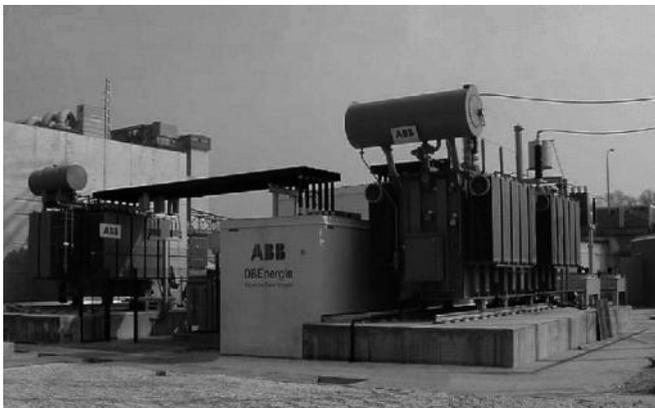
Fig. 13.8b: 15-MW standard railway supply converter (ABB Switzerland AG)
