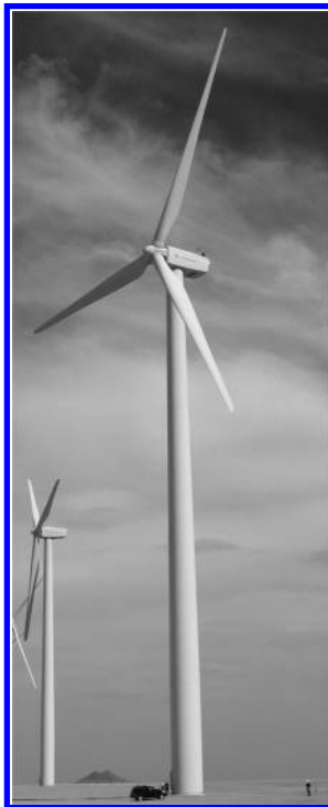
FIGURE 43.5 G.E. 1.5 MW wind turbines near Lamar, Colorado.
