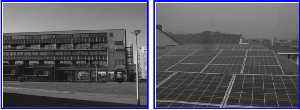
FIGURE 14.5 Building-integrated photovoltaics in a façade and in a roof.
