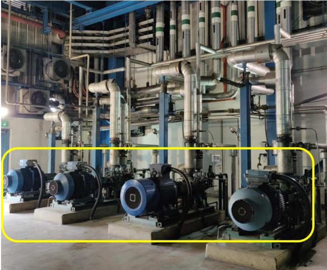
Figure 3.2 The actual LPFW motor on site at the CCPP
