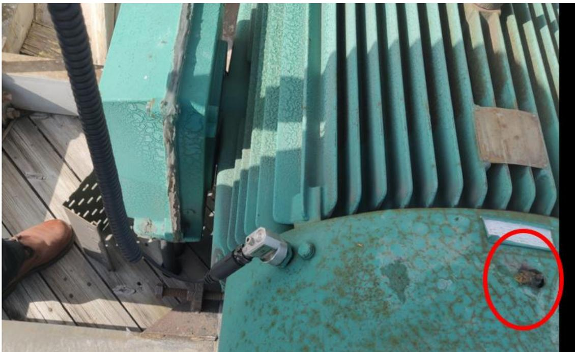
Figure 4.7 Shows sample electrical motor greasing point
