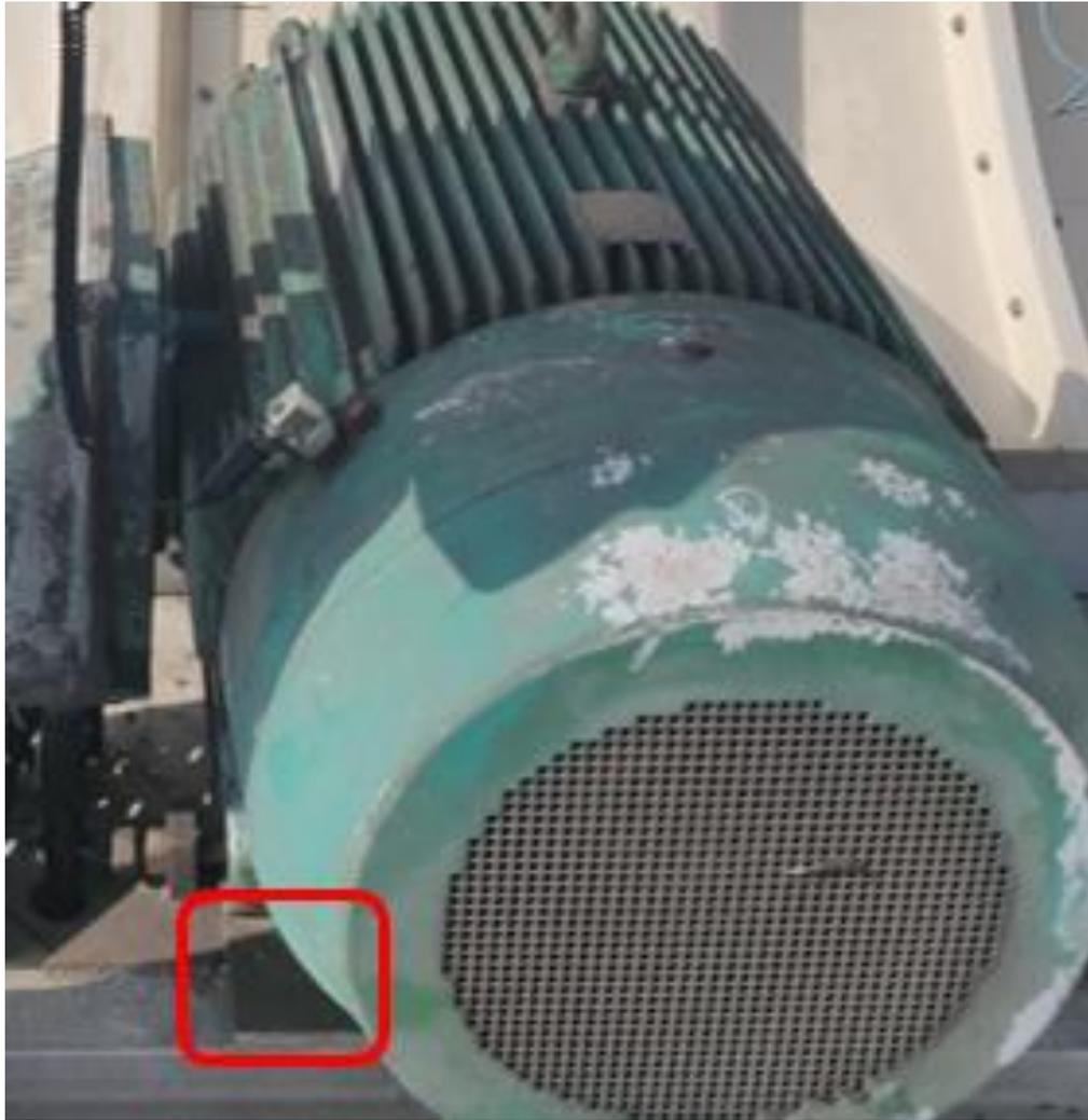
Figure 4.19 CT Fan Motor Base Frame Shim Replaced
