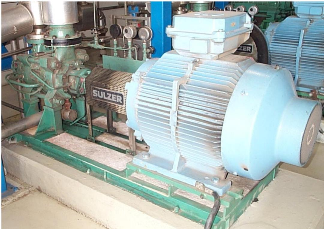
Figure 3.8 The LPFW pump motor no.4
